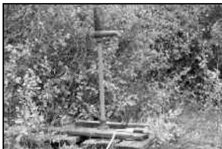
A well may provide a direct path for contamination to travel from the surface to the aquifer.
