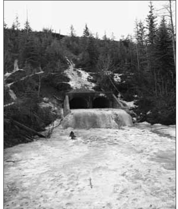
Canadian National Railways culvert on Hardisty Creek after remediation.
