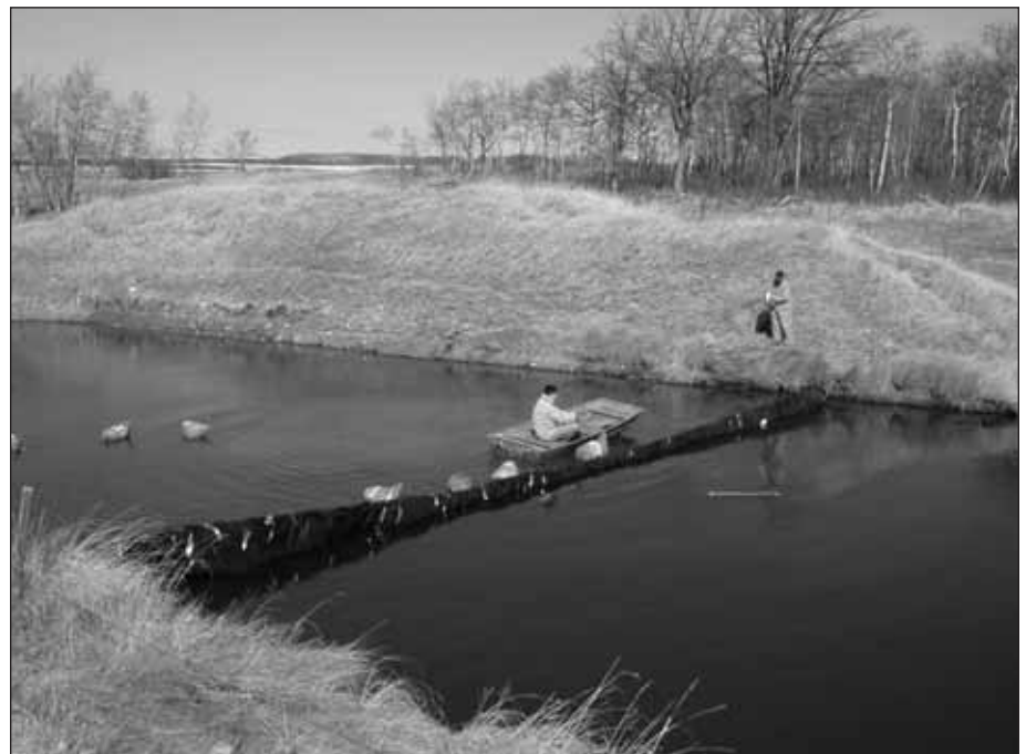
Typical dugout site showing geotextile membrane curtain and barley straw bags.
