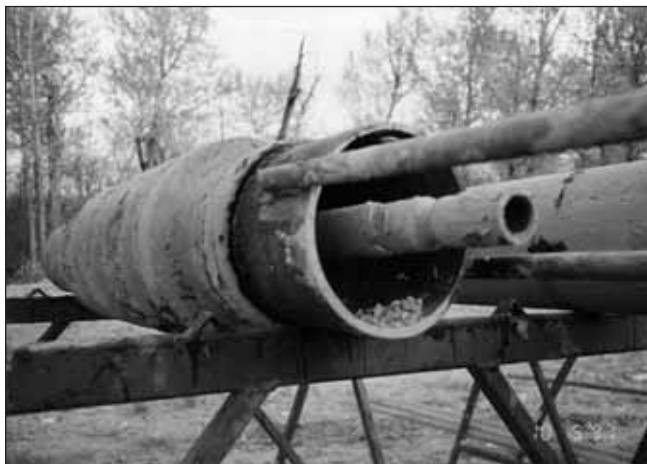
Biofilm encrustation on pump.
