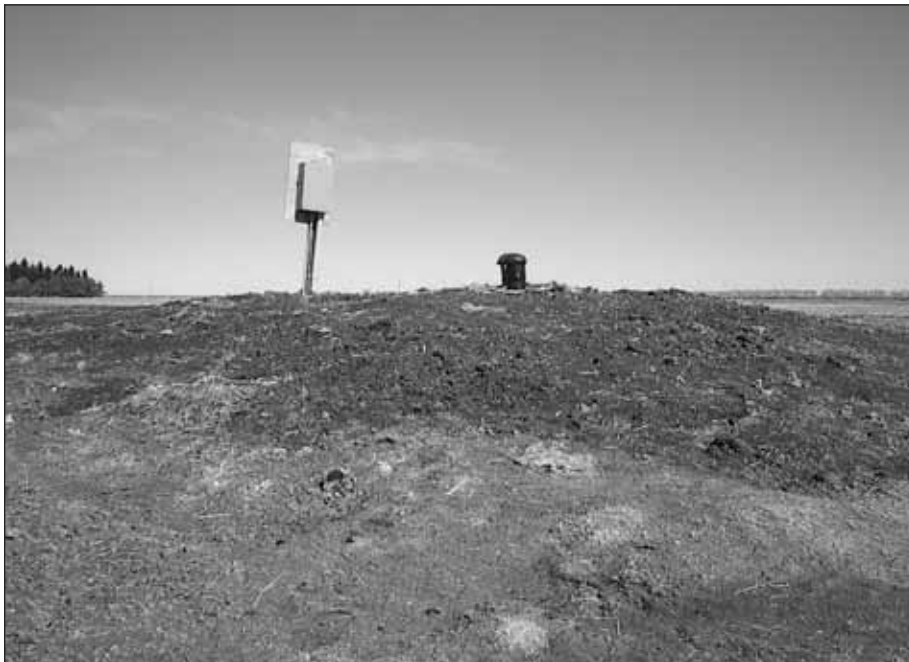
A well should always be built up with good clay to prevent any surface water from draining down the outside of the casing.
